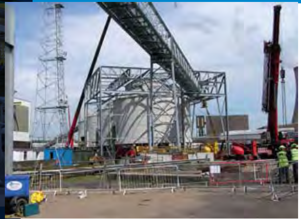
▲ A 4,000 MW Drax coal-fired plant in the United Kingdom includes storage silos for biomass pellets.
