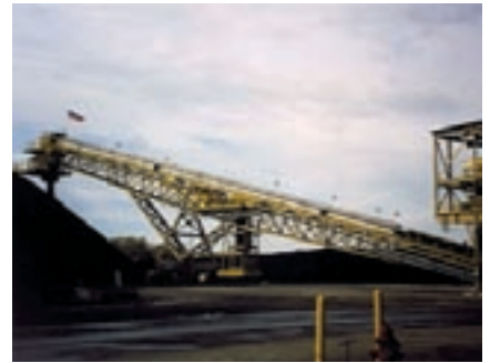
Fig. 5: The plant stacker unloading a trainload of PRB coal
