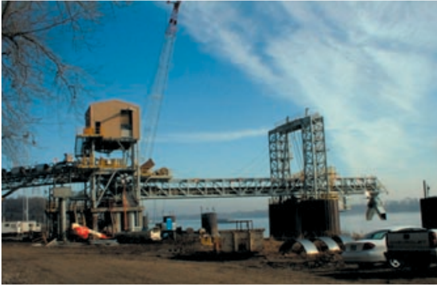
Fig. 8: Barge loader under construction
