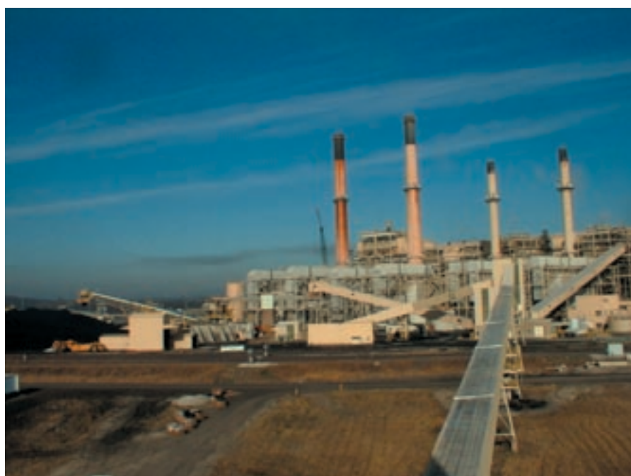
Fig. 1: The Meramec plant
