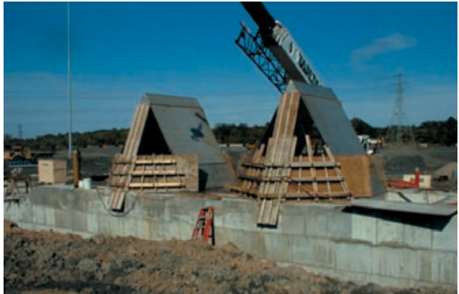
Fig. 6: Canopies being constructed at the reclaim belt feeders
