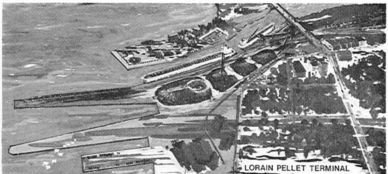
Fig. 3—Artist's rendition of Lorain pellet terminal developed by Republic Steel to reduce transportation cost. The facility accommodates 1000-ft. self-unloaders, stores pellets, and loads both river vessels and rail providing an economical and flexible transportation system.
