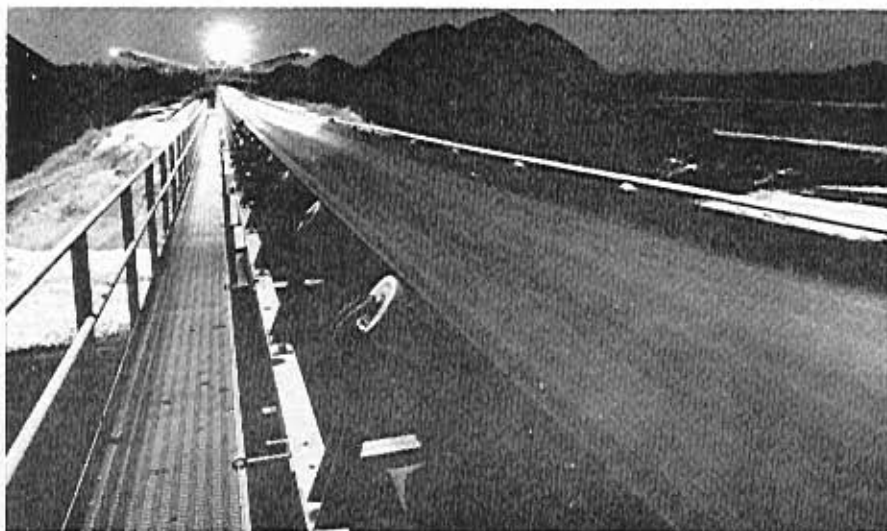
Fig. 1—Pride Transloader is a processor terminal situated in Pride, Ala. It receives and blends high, medium and low sulfur coal to provide Georgia Power with an environmentally acceptable and economical fuel. The different coal piles can be seen in the evening view of the stockpile and stacker.
